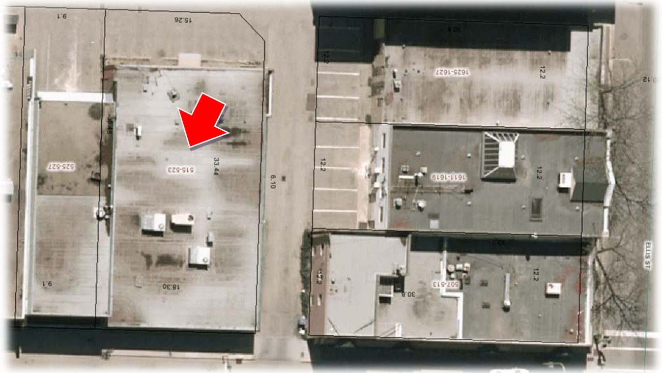
Aerial view showing building
